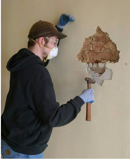
Left: Jessie begins slow process of exposing the brick walls.
