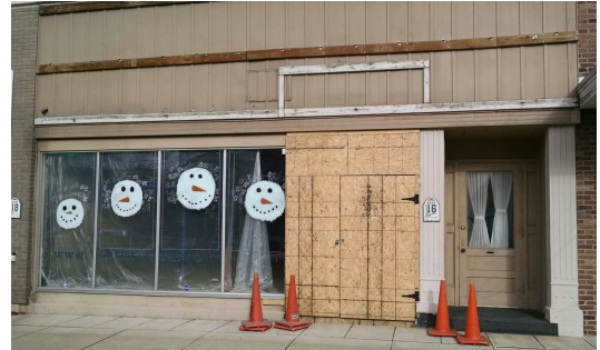
Facade redo in the works
